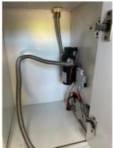
Make sure all the wires from the battery are connected. There are two switches. The top one is for the water pump to get water from the container to the sink; the bottom switch is for the freezer.
